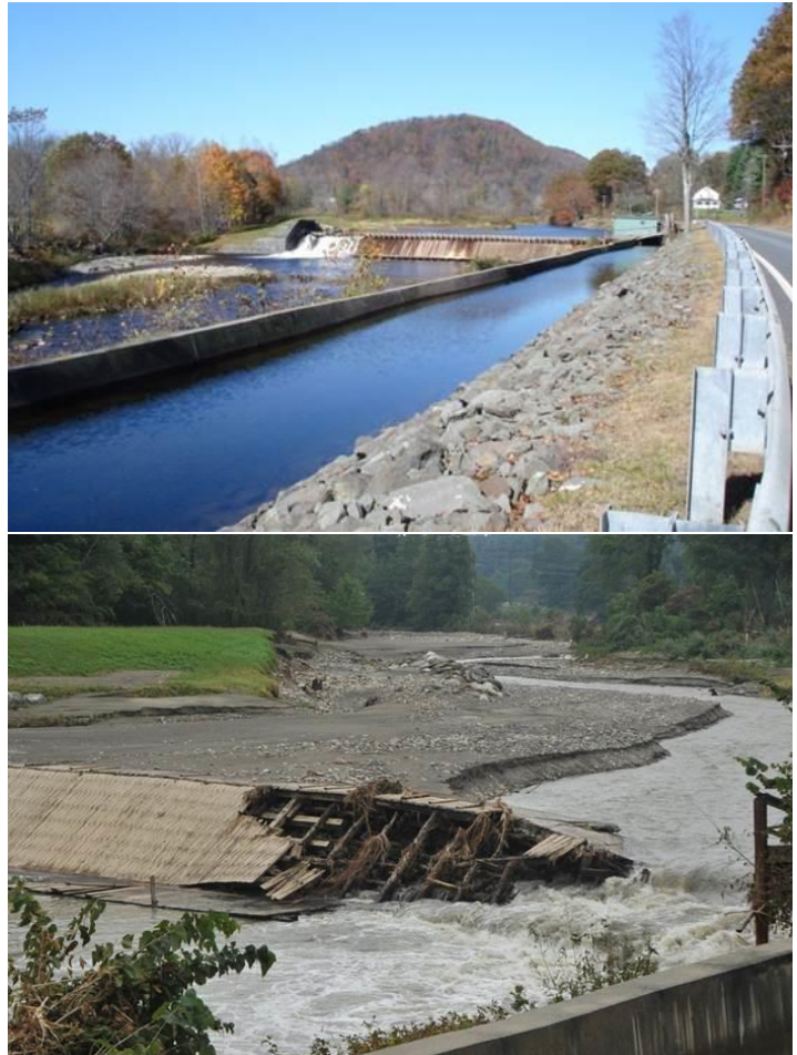
The East and West Branches of the North River have been subjected to flooding, including the washing away of a dam and riverbanks during Tropical Storm Irene. Top photo is before Irene; bottom photo is after.
