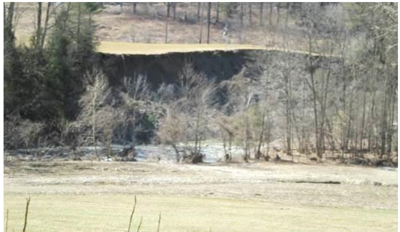
A large landslide on the East Branch of the North River is just one of many riverbank issues that exist on both branches of the North River in Colrain.
